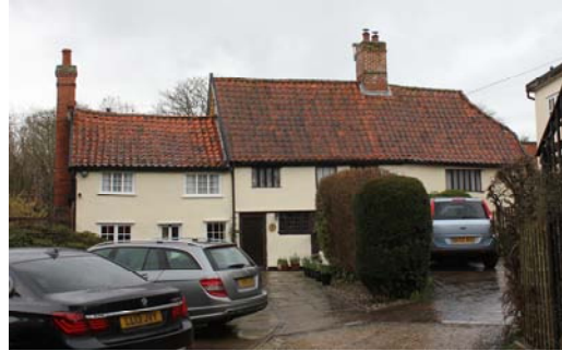
Fig 1: East front of 37-39 Church Hill
