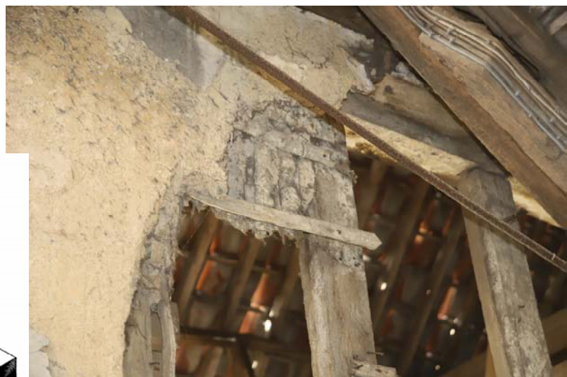
Fig 4: Exterior of east end of south wall of 17th C barn
