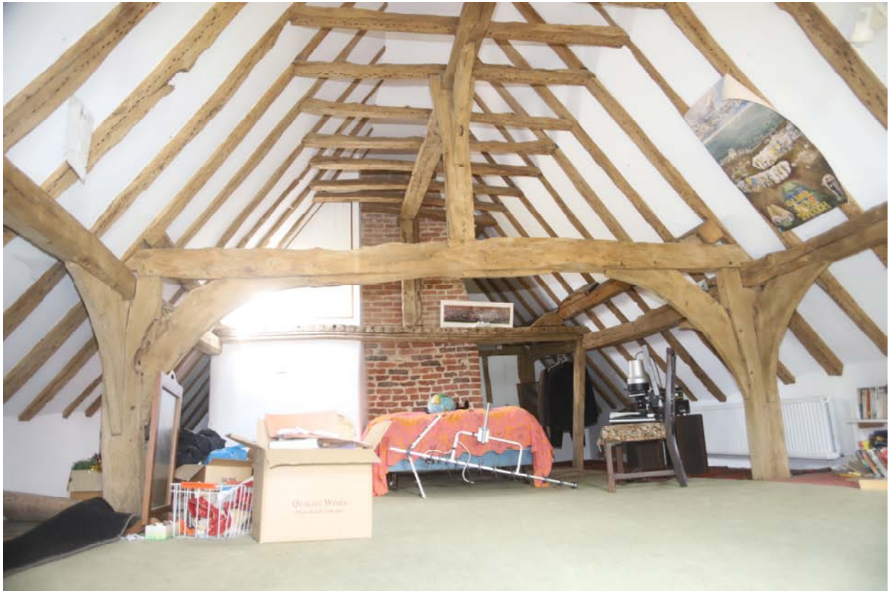
Two tier queenpost roof with crownpost above looking east to inserted chimney
