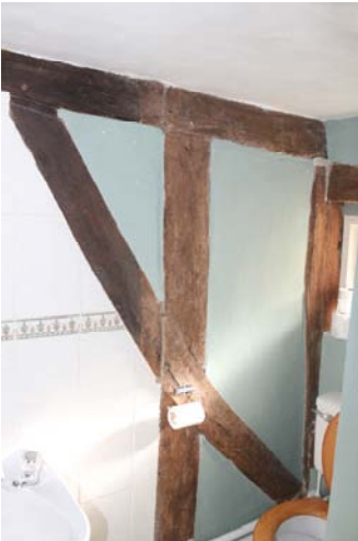
Fig 5: Jowled principal posts & drooping arch bracing in the south end wall
