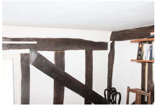
Fig 4: Close studding in the front wall of the hall chamber
