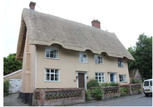
Fig 1: East front of 54 (left side) & 53 Low Street
