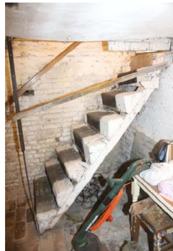
Fig 10: Reused solid stairs down into cellar under service rooms
